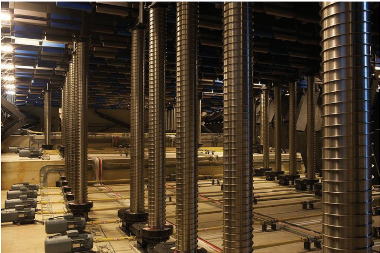
Detail of the Spiralift system beneath the seating platforms. • Credit: Hugo de la Morena
